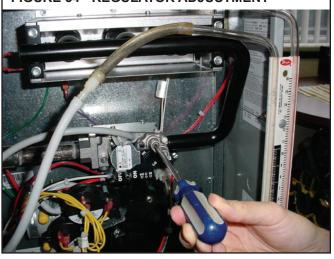
When the correct pressure has been established, securely replace the regulator cover screw.
