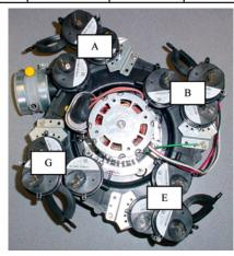
**EXAMPLE:** In a Horizontal Right/Vertical application (not shown), when the furnace is horizontal, room air is exiting from the right side of furnace, and the flue is vertical (exiting from the left side panel in an upflow position), the pressure switch should be mounted at location A or E.
