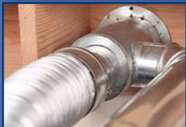
Flexible Vent Pipe
