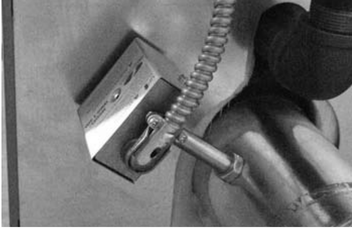
Figure 3 - Acceptable Mounting Position 1
