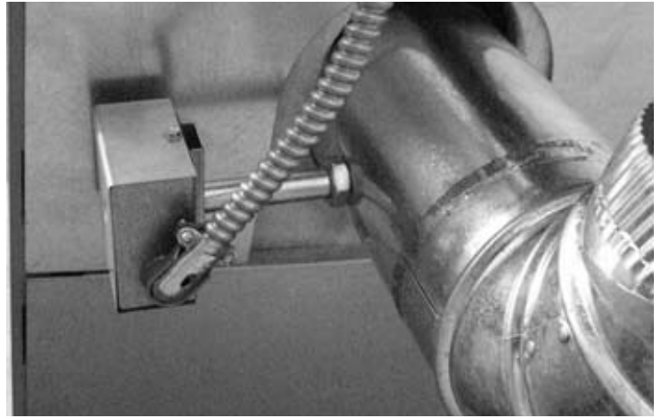
Figure 4 - Acceptable Mounting Position 2
