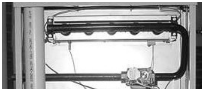
Figure 24- Inshot Burner Assembly
