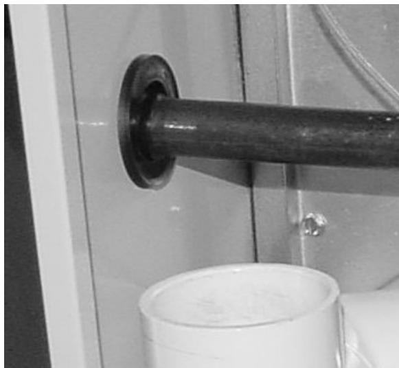
Figure 23 - Furnace Gas Pipe Connections (Note Rubber Grommet)
