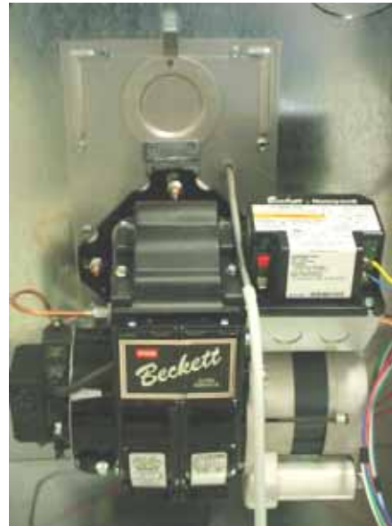
Fig. 1: Checking Over-Fire Draft.
