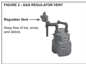
It is important for these vents to remain clear. Do not allow moisture, which could freeze, to build up in the vent. If you see moisture building up in the regulator vent, contact your gas supplier.
